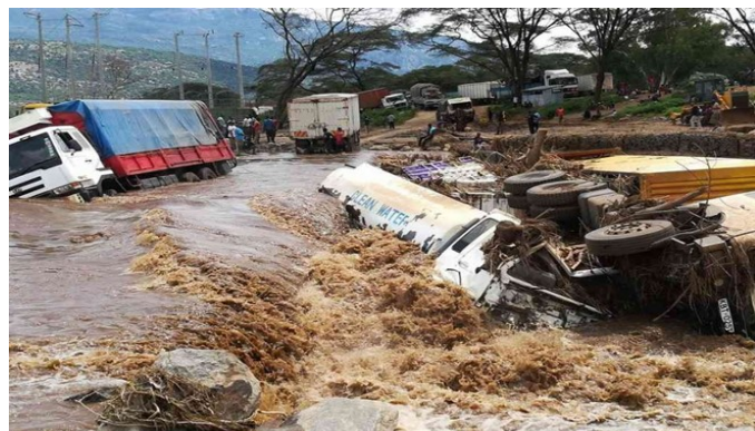
Plate 1: Flooding and damage at Kainuk Bridge in Turkana County. (Source: KeNHA, 2018).
