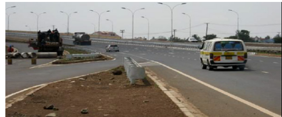
PLATE 1 Insufficient weaving length Source: Field survey 2015
