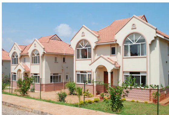
FIGURE 17 Contemporary houses in Uganda Source: Wambui 2011
