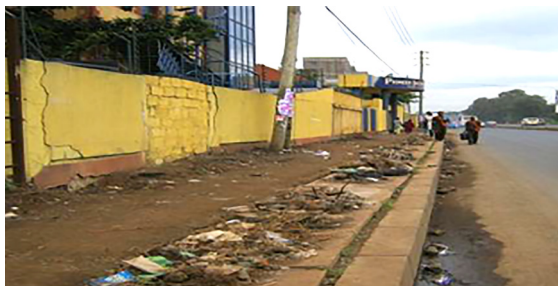
PLATE 4 Carriageway along Muthaiga Roundabout to Uhuru Highway zone Source: Field survey 2015
