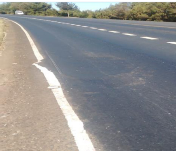
6c) Pothole cluster in the transition zone between steep and rolling terrain
