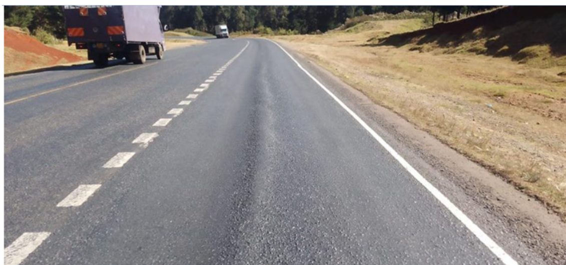
6e) Rutting along the climbing lane section
