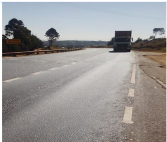
6d) Rut formation along the climbing sections
