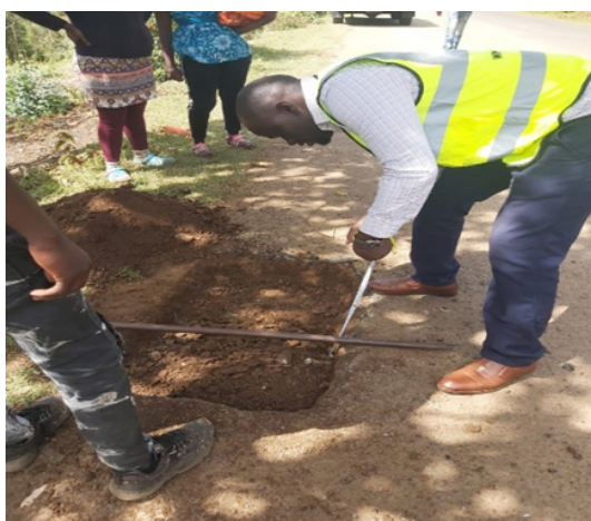
b) Surfacing thickness measurement
