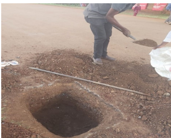
a) Sampling of excavated pavement material
