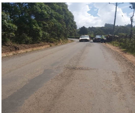
a) Intact section with lined drains at km 2.3
