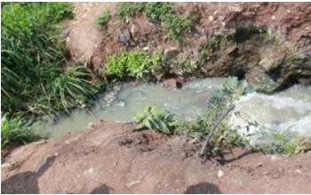
FIGURE 12 Sewer from apartments in Ngara draining into the Nairobi River Source: Field survey, 2025
