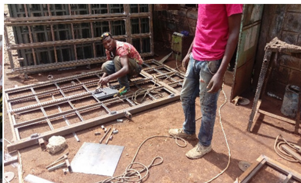
FIGURE 9 Industrial-oriented activity (welding) Source: Survey (2020)
