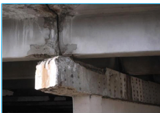
FIGURE 1 (a) Damage due to corrosion for non-integral bridges Source: Martin.et.al, (2009)
