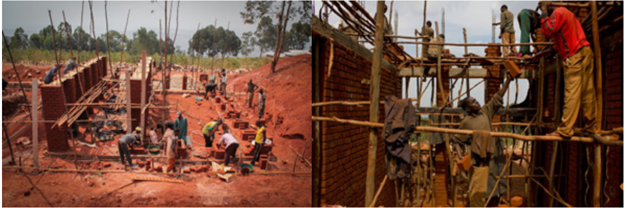
FIGURE 17 Building from nature, construction works in progress Source: BC Architects, 2012
