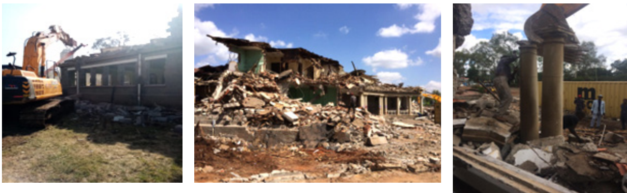
FIGURE 7d Structure demolition Source: Authors 2020
