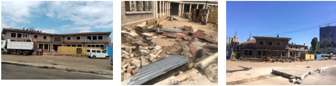
FIGURE 7b Pitched roof demolition Source: Authors 2020
